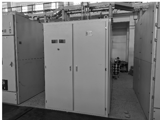
图10 大功率电弧加热器电源 Fig. 10 Power supply for high-power arc heater
